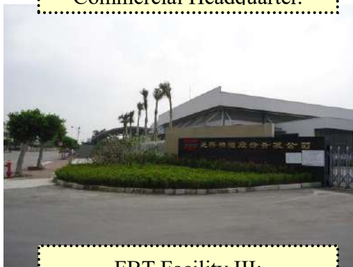
FBT Facility III: Disk & Production Center
